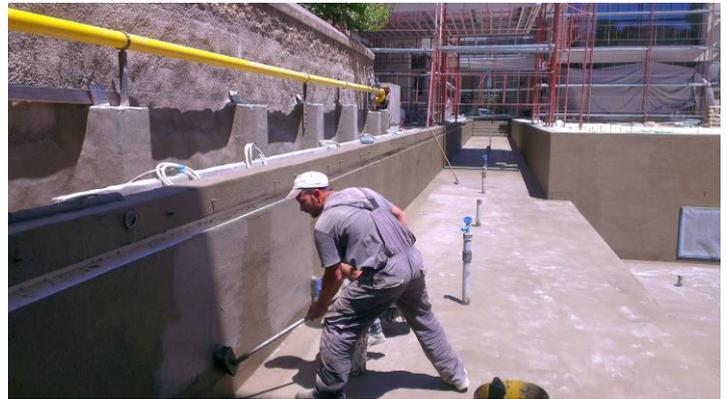
In order to place ceramic tiles on top of SEALCOAT™ SYSTEMS, use an appropriate FLEX type adhesive paste for pool application.
