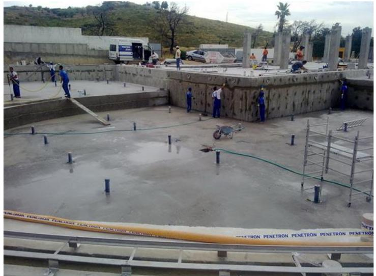
In the case of equipment installation or piping, after the pool construction, that need round sealing/waterproofing, the use of the appropriate circumferential application PENEBAR® SW is recommended (the recommended type is the control-expanding PENEBAR® SW 55 TYPE B or sometimes the half of the Type 55 B). PENEBAR® SW is placed in a depth at least approx. 2" (5 cm) and covered with the rapid-setting crystalline waterproofing plug PENEPLUG®.
